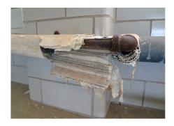
The area of damaged ACBM is repaired with such materials as asbestos-free spackling, plaster, cement, or insulation; sealed with latex paint or an encapsulant; or an appropriate response action is implemented as required by § 763.90 of the AHERA Rule
